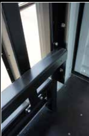
Frame adjustable in all directions.
