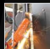
Quick saw & Chain Saw Breaching
